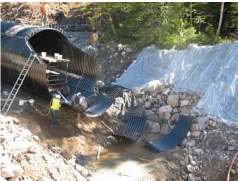
Figure 6. A corrugated metal pipe culvert being installed.
