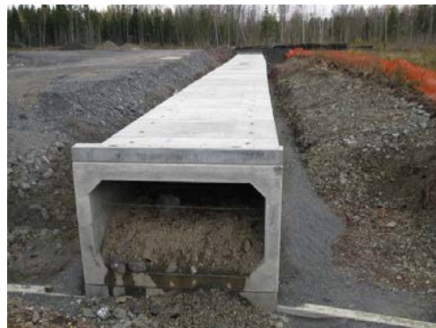
Figure 5. Example of an embedded culvert.
