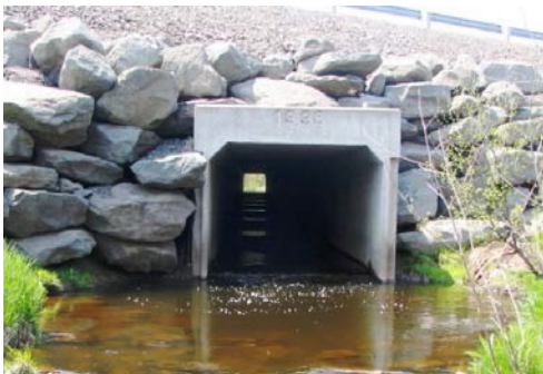
Figure 8. Example of a concrete box culvert.
