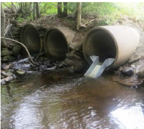
Figure 25. A chute installation on a culvert
