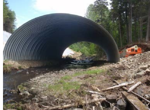
Figure 3. Example of a properly installed open-bottom structure.
